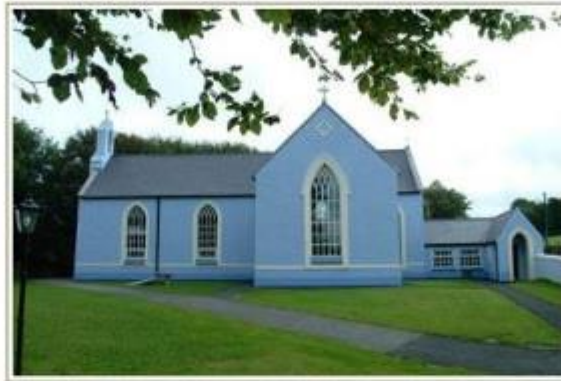
Minane Bridge Church
